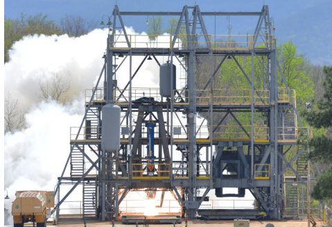
Rocket Test Center at Redstone Arsenal
